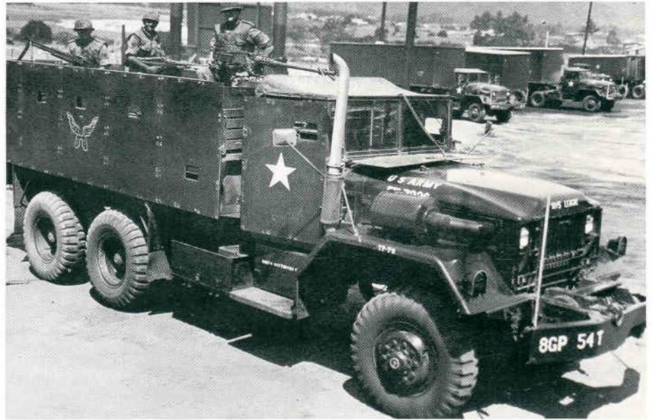
Five ton M-54 truck with 2 M-60s and a .50 caliber mount behind the cab. Though extremely helpful in convoy security each modified truck took away a needed cargo carrier and men from the overworked transport groups. (US Army)
