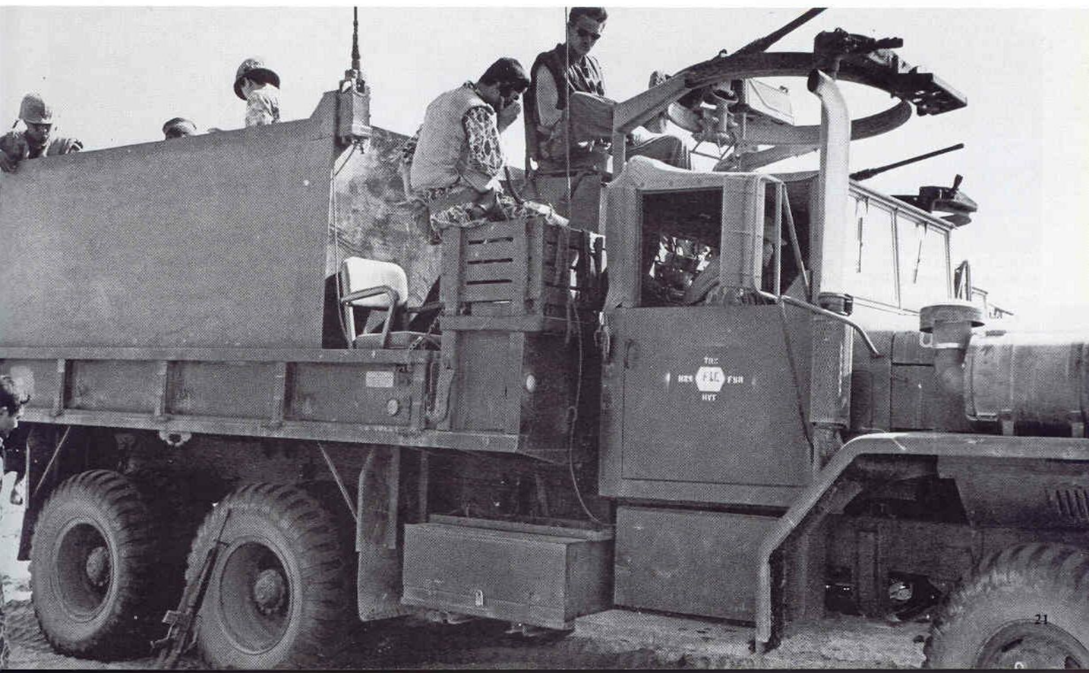
War Wagon , a five ton truck, one of a number which were armored to provide convoy security. Note variety of uniforms among crew. (USMC)
