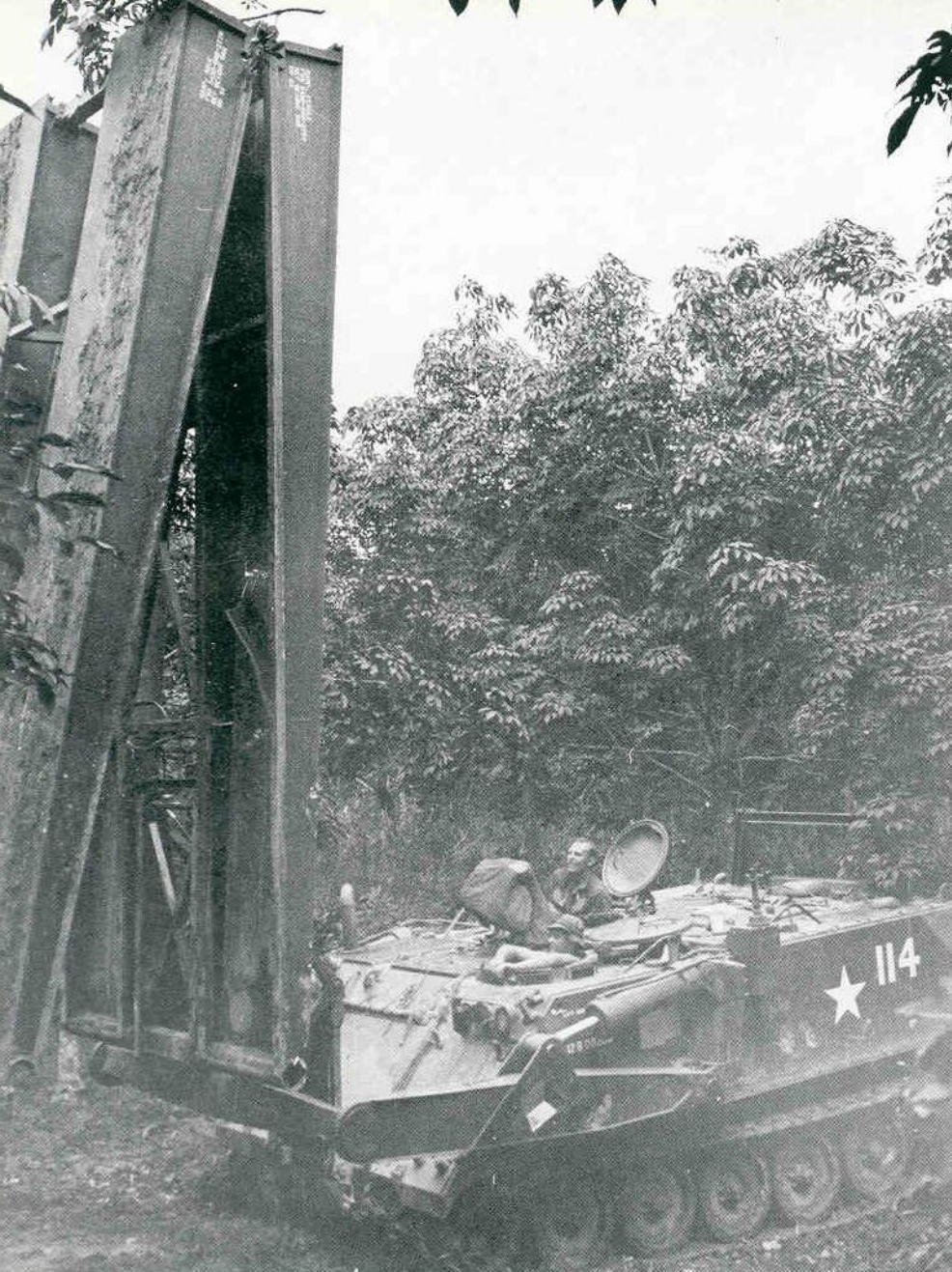
Bridgelayer M-113 picks up its span before moving on to another bridging operation. These vehicles provided a cheap, easy conversion and proved extremely valuable in helping span gullies and road cuts of under 30 feet. (US Army)
