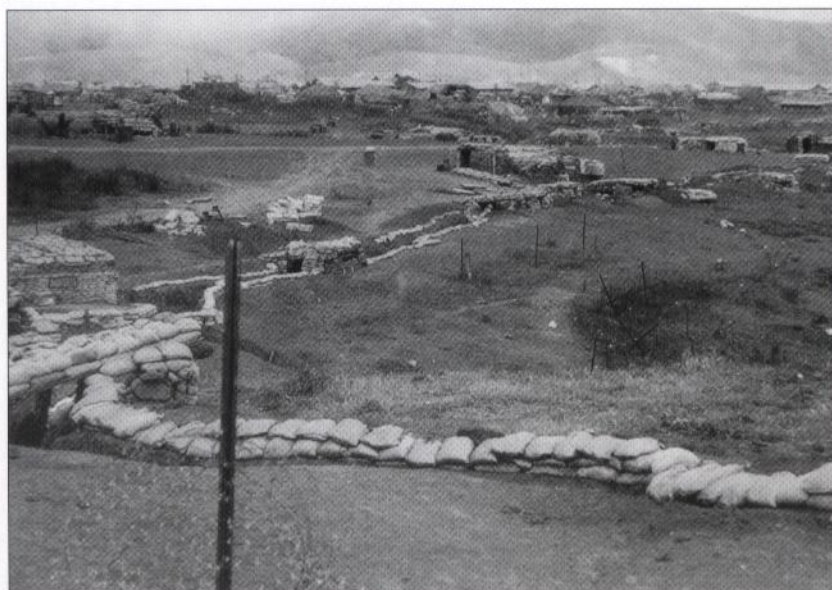
Cloud-shrouded hills provide the backdrop to KSCB. This is the north perimeter trench showing fighting bunkers along the trench line. The gray-green woven plastic and tan burlap sandbag parapets against the dark red soil highlight the trench outlines. The airfield is beyond the buildings and tents in the background.
