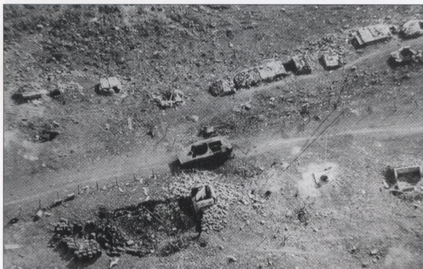
Lang Vei Special Forces Camp after its fall on February 7, 1968. In the center is the hulk of a PT-76 tank with its turret blown off. Immediately below it is the observation post bunker blasted by demolition charges and its sandbag revetting blown away. To the left of the OP bunker is the collapsed roof of the underground command bunker. The battered 55gal drum barricade can be seen at the command bunker's left end. The south perimeter fighting bunkers of the central position can be seen above the carnage of the command bunker.
