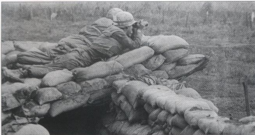
A pair of Marines lay atop their perimeter bunker searching for the faint telltale puff of smoke of a mortar firing. This was extremely difficult among the vegetation, dust, and fog. The three-sandbag-thick roof is laid atop recovered M18 airfield matting. Draped over the sandbags are firing wires leading to M18A1 Claymore antipersonnel mines in the barrier wire.
