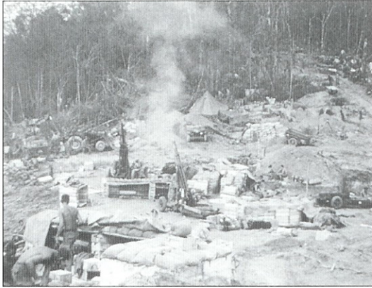
A firebase hacked out of the jungle was in a constant state of construction. Sandbags, empty ammunition boxes, and pallets were the basic construction materials for fighting positions, bunkers, and living quarters, called "hooches" regardless of the form they took. Here a battery of 105mm M102 howitzers is being emplaced.
