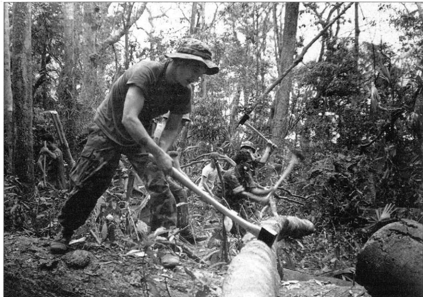
Groundwork included clearing trees and vegetation to allow helicopters to bring in engineer support and material to rapidly bring the fire support base into operation. The initial landing zones were levelled with hand tools. (DOD)
