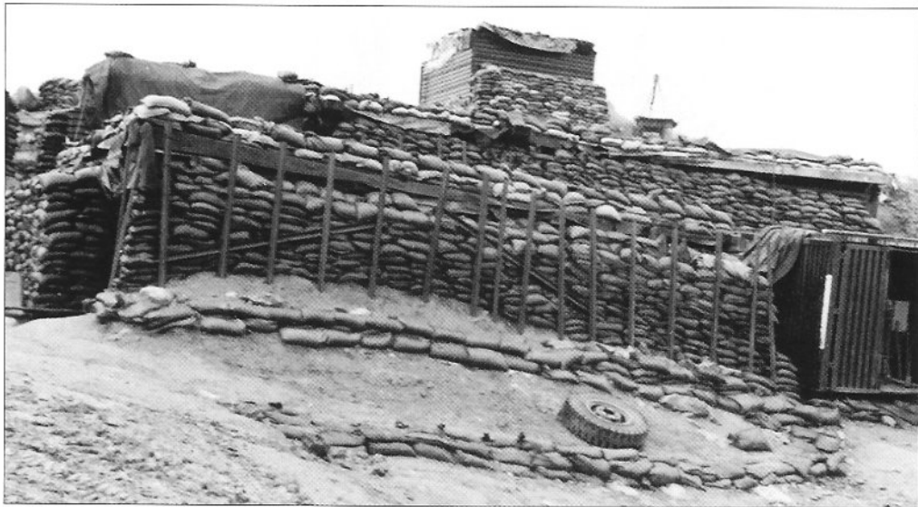
A large, sandbagged bunker complex used as living quarters at FSB Anzio, Thua Thien province, incorporating a steel Conex box at bottom right. (US National Archives)
