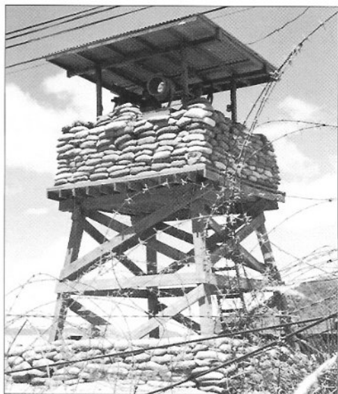
A well-constructed timber-framed observation tower for a searchlight, including corrugated steel roof and plentiful sandbags. Presumably an underground bunker would be at its base (1st Bn, 21st Artillery, 1st Air Cavalry, May 1967). (US National Archives)
